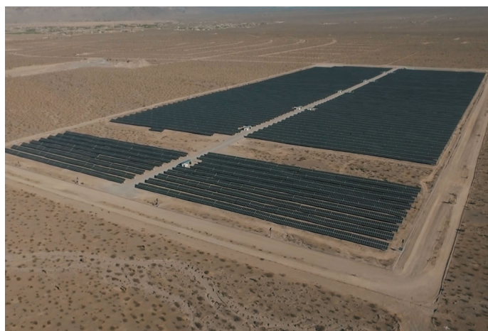
The 15 MW utility-scale solar array in Pahrump that Bombard completed for the Valley Electric Association covers 80 acres, includes 50,000 panels (all made in the U.S.A.) and helps protect habitat for desert tortoises. (Photo courtesy of Bombard)
